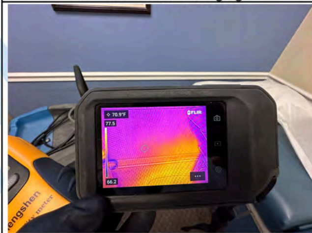
Room 3 - Thermal Imaging
