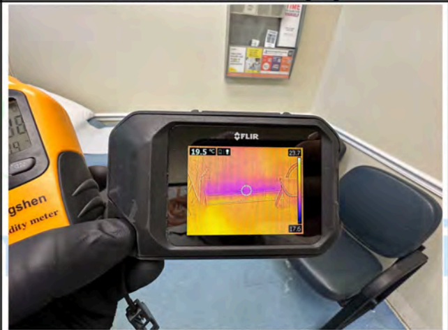
Room 2 - Thermal Imaging
