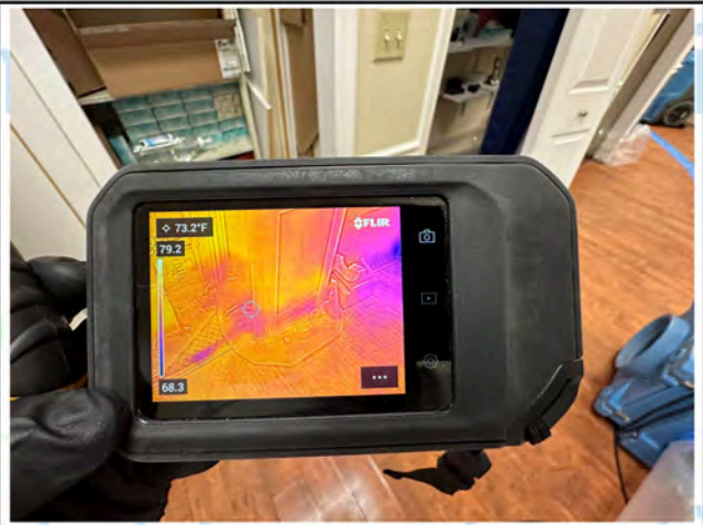
Main Hall 4 - Thermal Imaging
