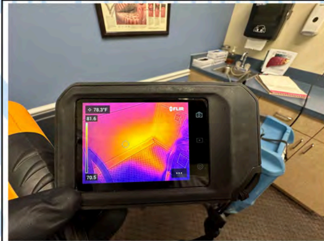
Room 4 - Thermal Imaging
