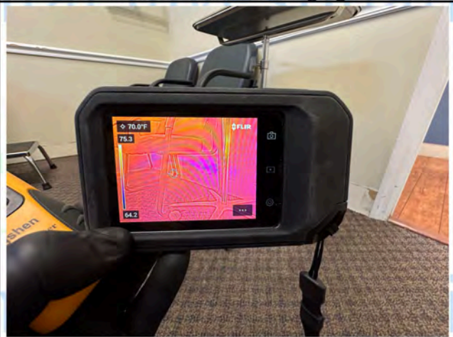
Room 3 - Thermal Imaging
