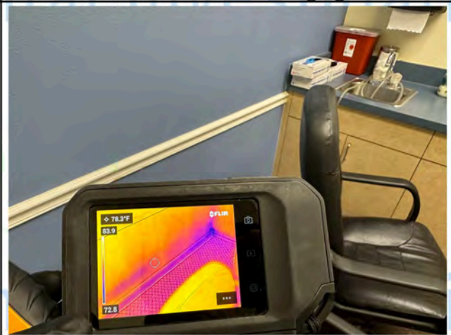
Room 5 - Thermal Imaging
