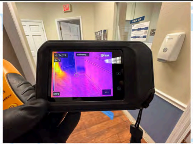
Main Hall 4 - Thermal Imaging
