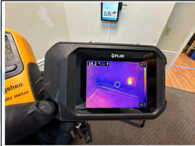
Room 1 - Thermal Imaging
