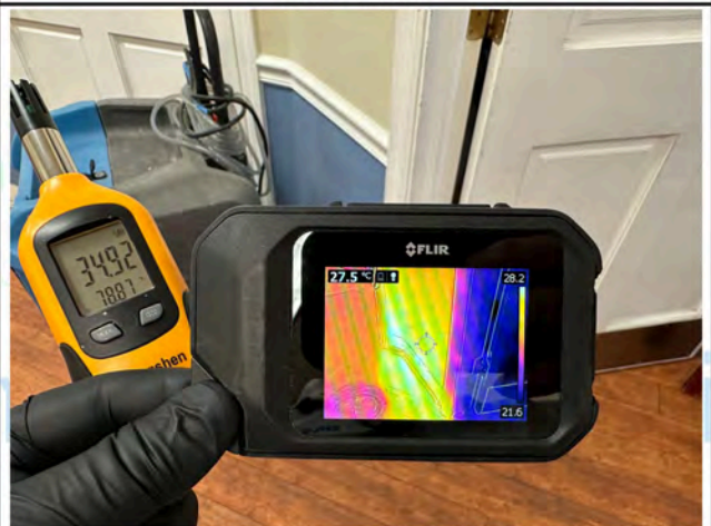
Main Hall 1 - Thermal Imaging
