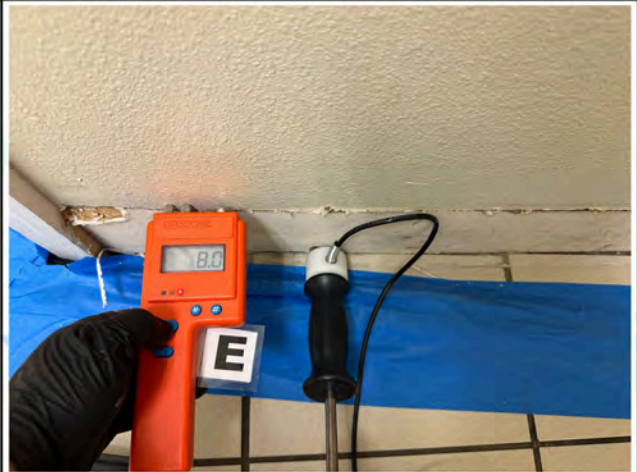
Women's Bathroom - Drywall
