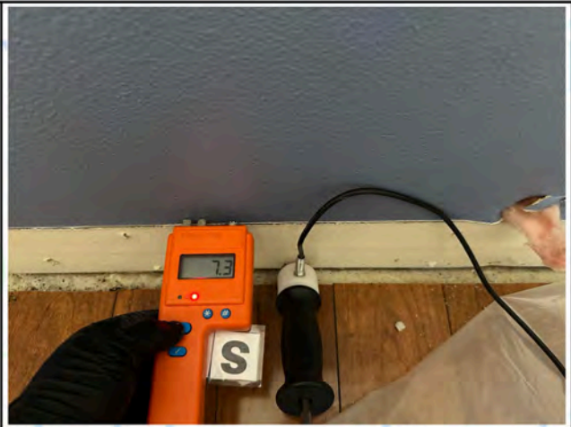
Waiting Room - Drywall
