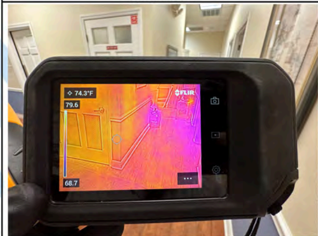
Main Hall 3 - Thermal Imaging
