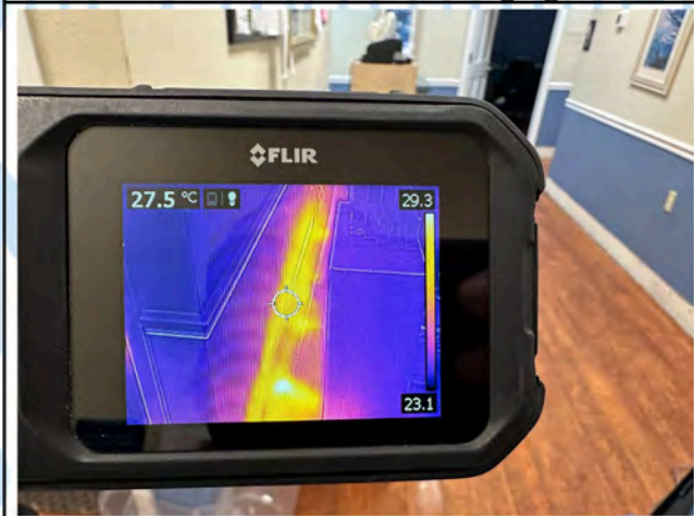
Main Hall 1 - Thermal Imaging
