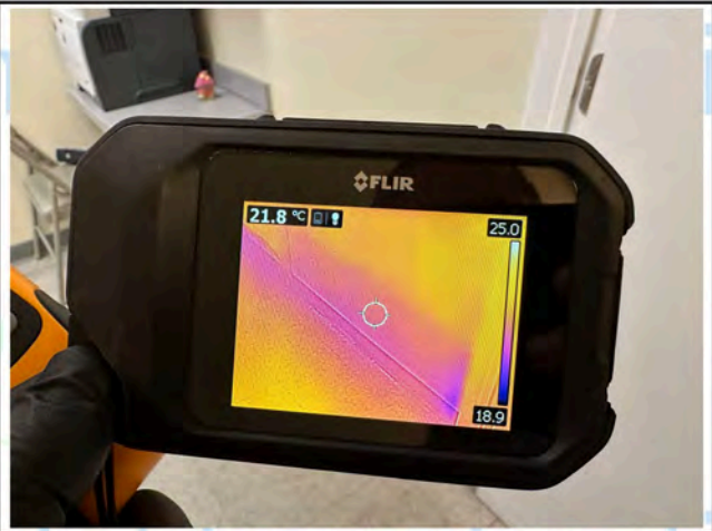
Office 4 - Thermal Imaging
