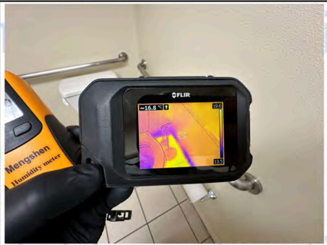
Women's Bathroom - Thermal Imaging
