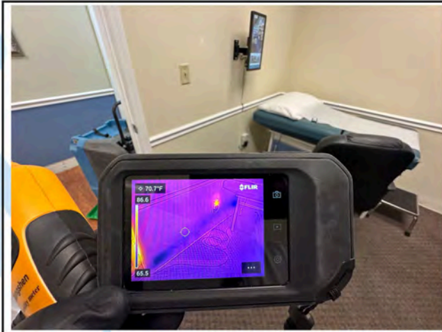
Room 4 - Thermal Imaging
