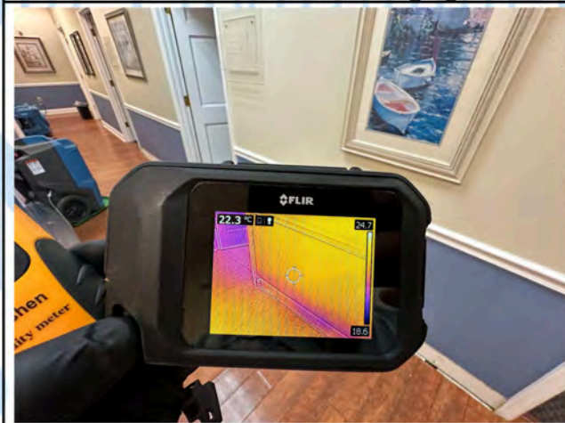
Main Hall 2 - Thermal Imaging
