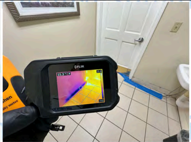
Women's Bathroom - Thermal Imaging
