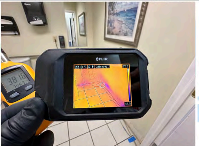
Men's Bathroom - Thermal Imaging
