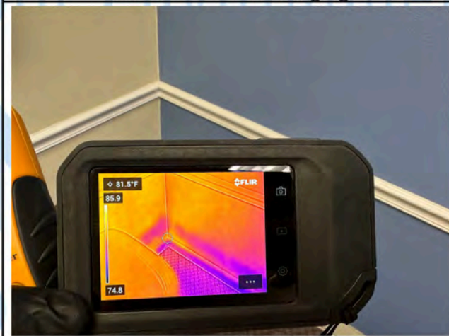
Room 5 - Thermal Imaging
