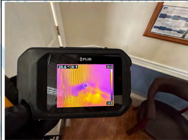
Waiting Room - Thermal Imaging
