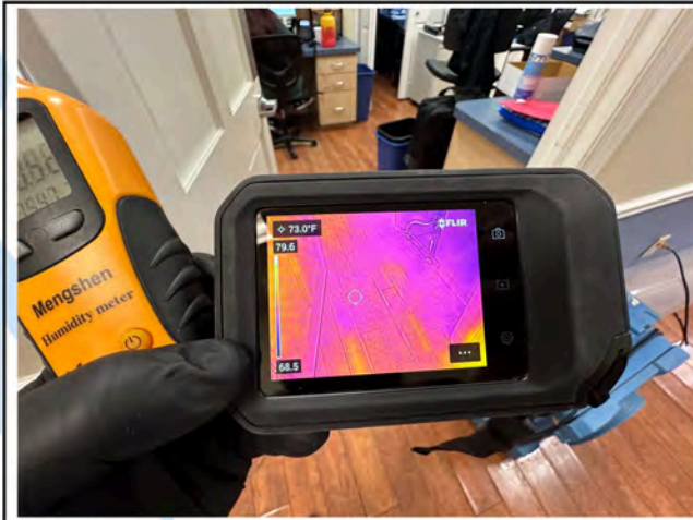
Main Office - Thermal Imaging
