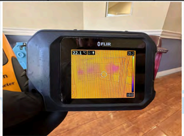
Waiting Room - Thermal Imaging
