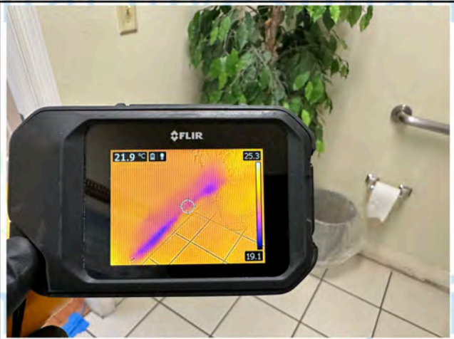
Men's Bathroom - Thermal Imaging
