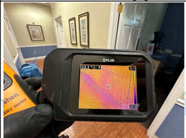
Main Hall 2 - Thermal Imaging
