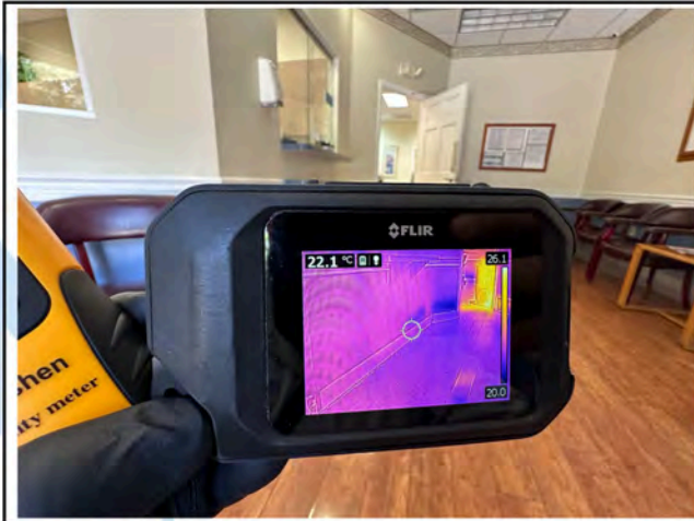
Waiting Room - Thermal Imaging
