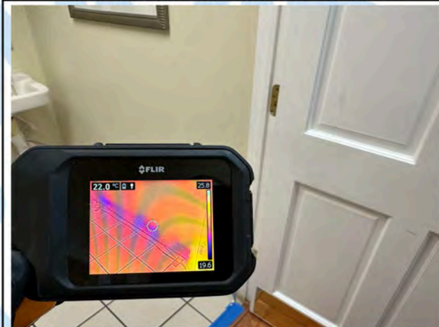
Men's Bathroom - Thermal Imaging
