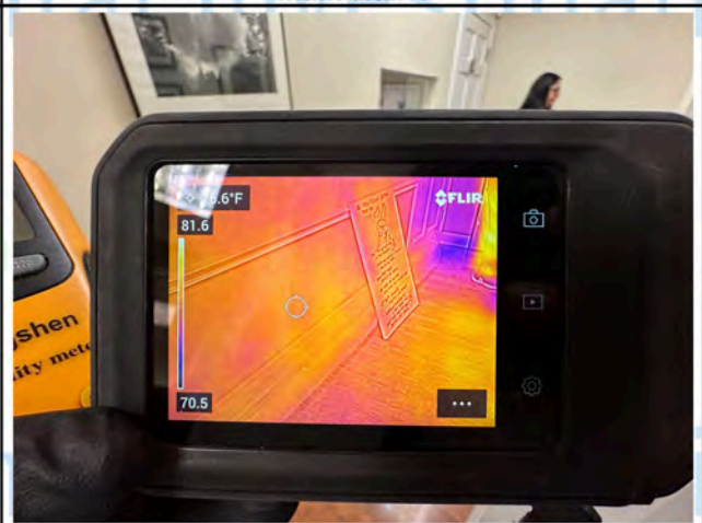
Main Hall 4 - Thermal Imaging
