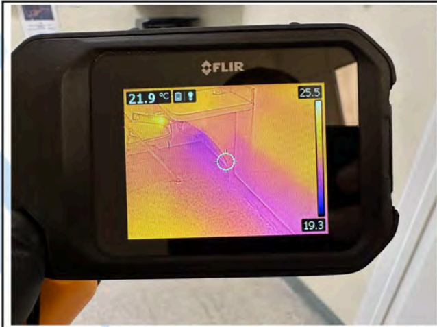
Office 4 - Thermal Imaging
