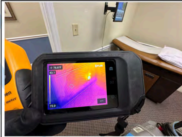
Room 5 - Thermal Imaging
