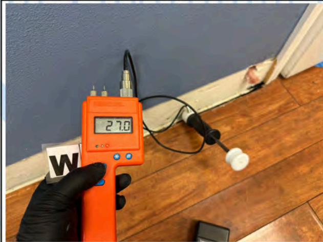
Main Hallway 1 - Sill Plate
