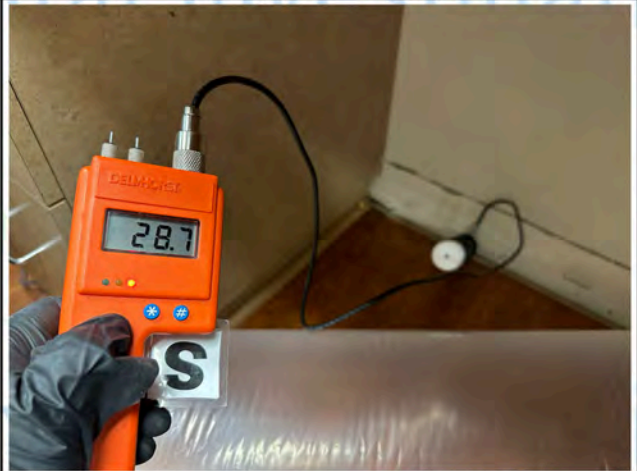
Main Office - Sill Plate
