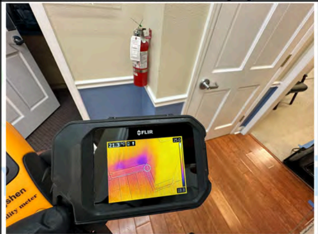
Main Hall 2 - Thermal Imaging
