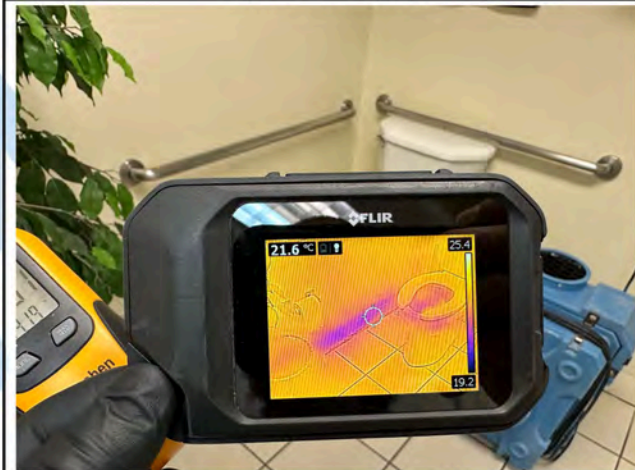
Men's Bathroom - Thermal Imaging
