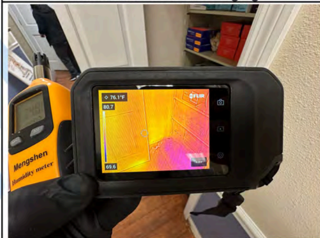
Main Hall 4 - Thermal Imaging
