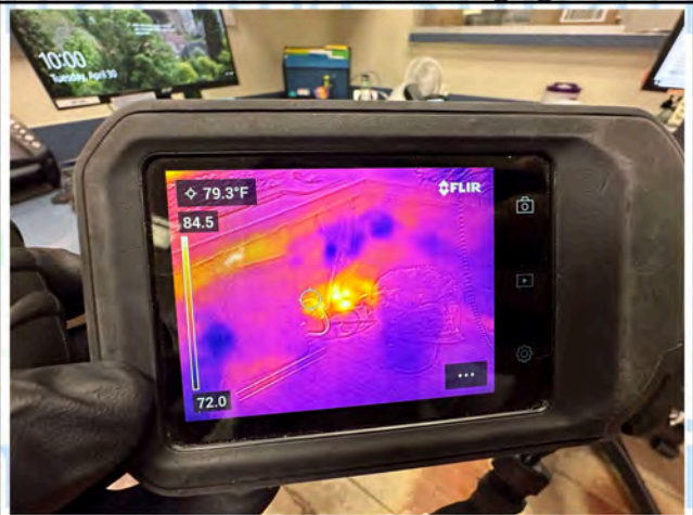
Main Office - Thermal Imaging
