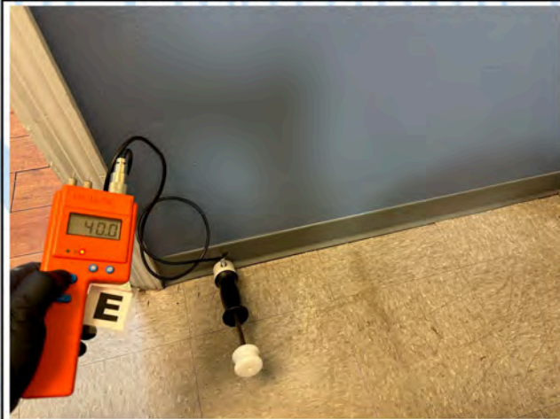
Hallway 1 - Sill Plate
