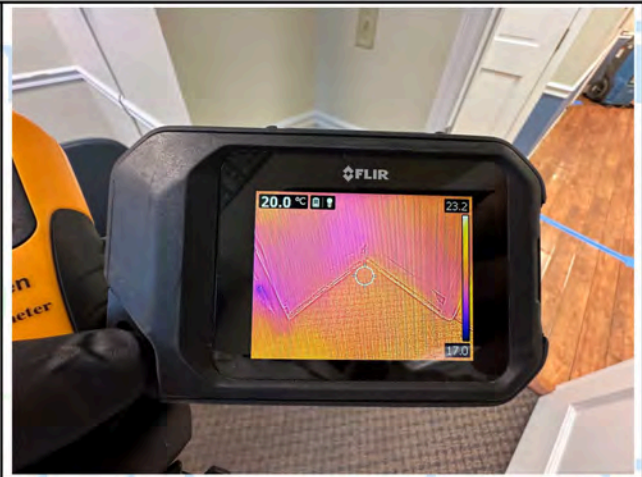
Room 1 - Thermal Imaging
