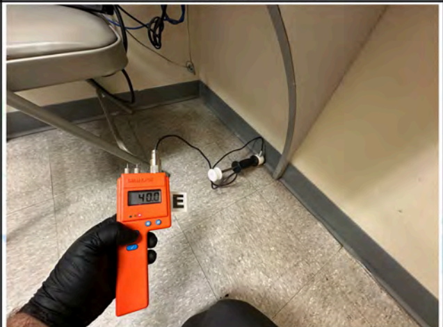
Office 4 - Sill Plate
