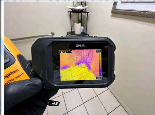
Women's Bathroom - Thermal Imaging
