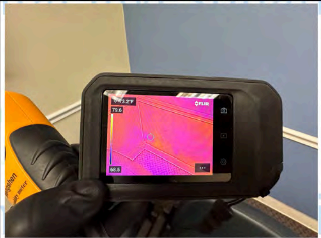
Room 4 - Thermal Imaging
