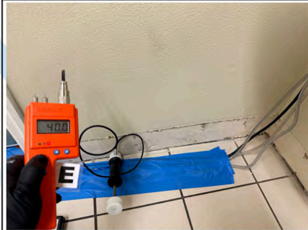
Women's Bathroom - Sill Plate
