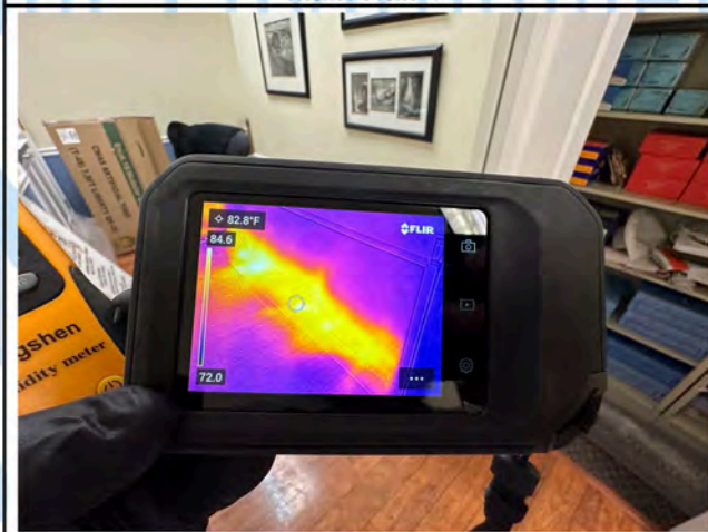
Main Hall 4 - Thermal Imaging
