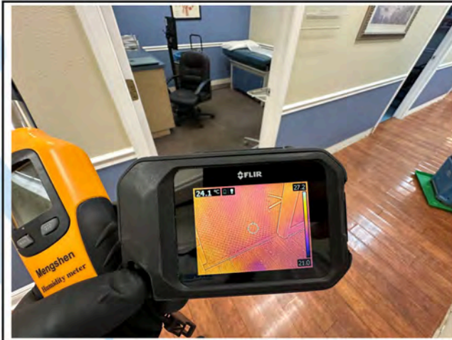
Room 3 - Thermal Imaging
