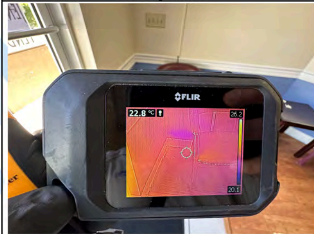
Waiting Room - Thermal Imaging
