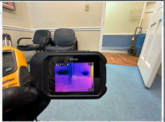
Room 2 - Thermal Imaging
