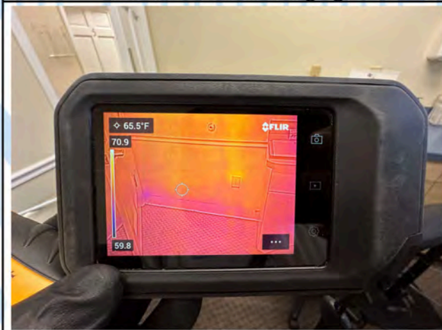
Room 3 - Thermal Imaging
