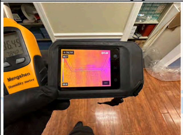
Main Hall 4 - Thermal Imaging
