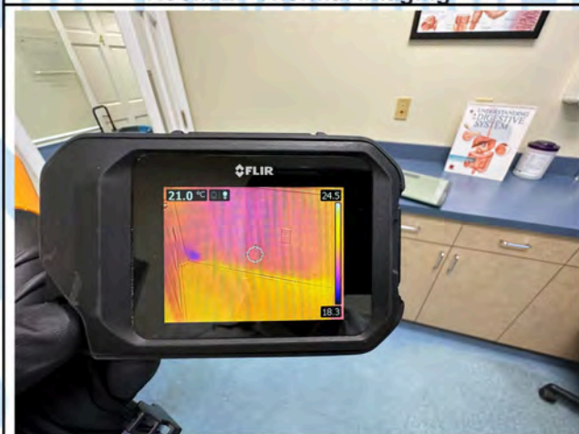
Room 2 - Thermal Imaging
