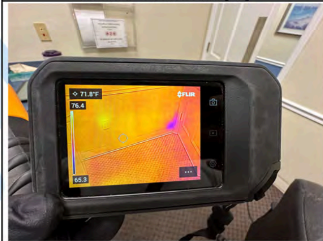
Room 4 - Thermal Imaging
