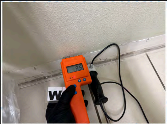
Men's Bathroom - Drywall
