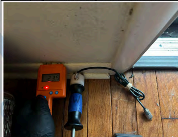
Drying Station Living Room - Drywall
