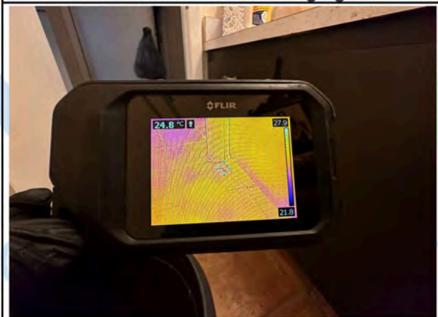
Bathroom Thermal Imaging
