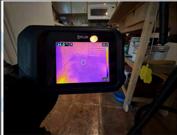
Kitchen Thermal Imaging
