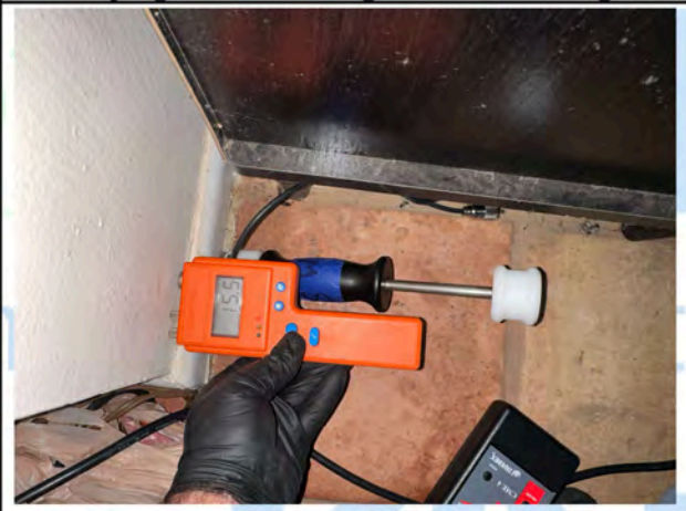
Drying Station Dining Room - Drywall
