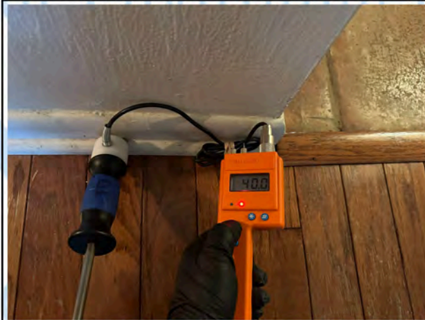
Drying Station Living Room - Sill Plate
