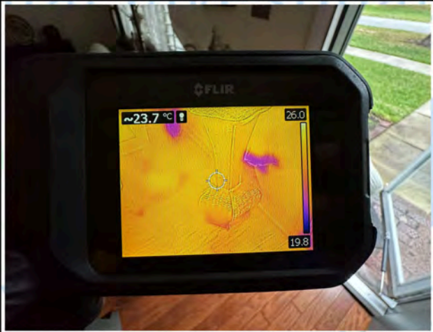
Living Room Thermal Imaging
