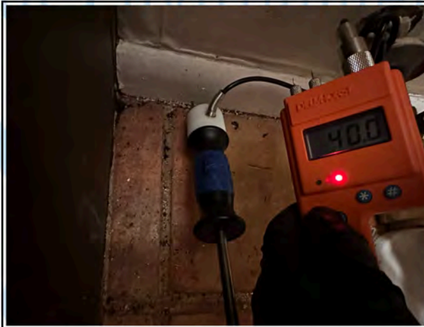
Drying Station Bathroom - Sill Plate
