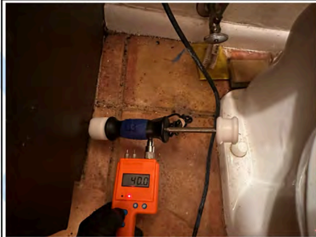
Drying Station Bathroom - Vanity
