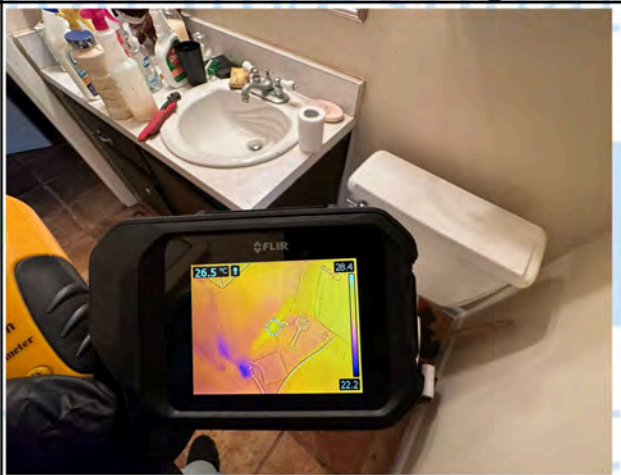
Bathroom Thermal Imaging
