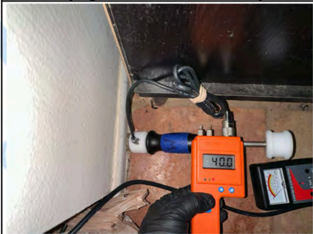
Drying Station Dining Room - Sill Plate
