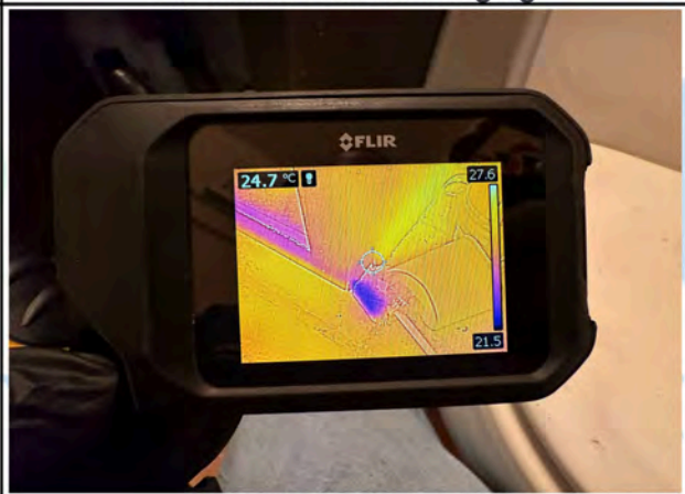
Bathroom Thermal Imaging
