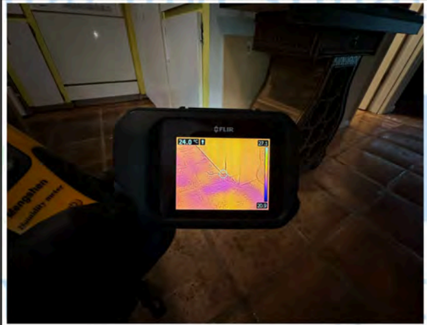
Kitchen Thermal Imaging
